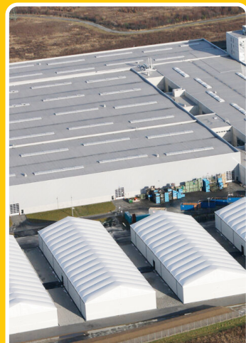
6. Professional Industrial Structure Installation
