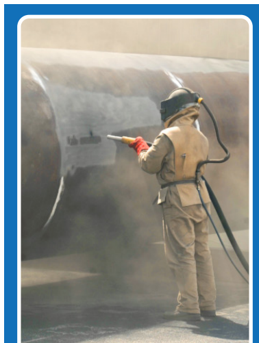
5. Pipe and Crossover Sandblasting and Cleaning
