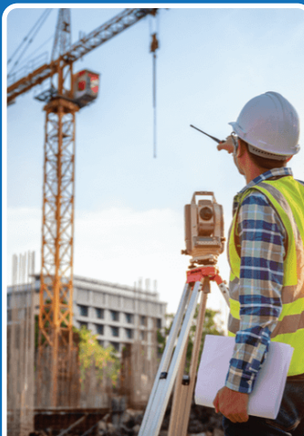
5. Rigorous Structural Inspection and Maintenance
